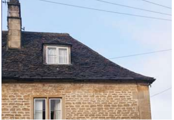
Slight eaves 'bell cast'
