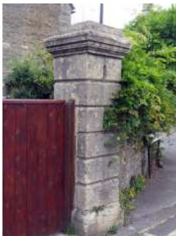
Middlewick Lane gate pillar
