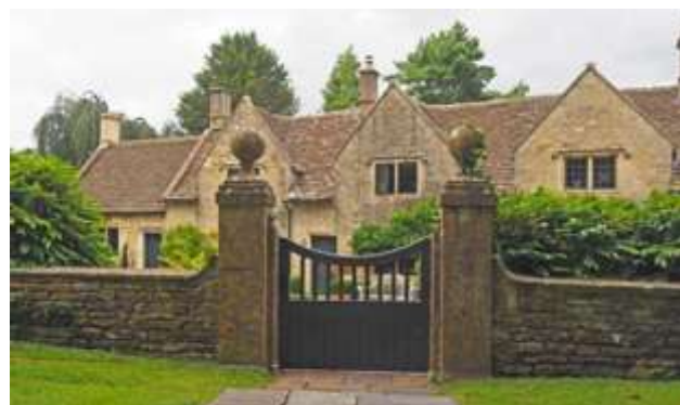
Hillsgreen Lodge at Upper Pickwick
