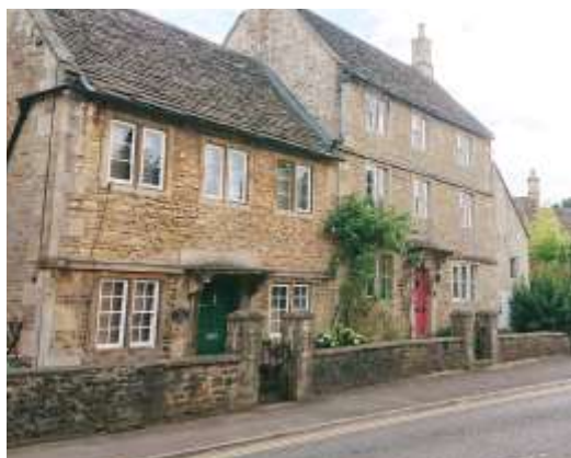
The listed low boundary wall at 20 and 22 Pickwick
