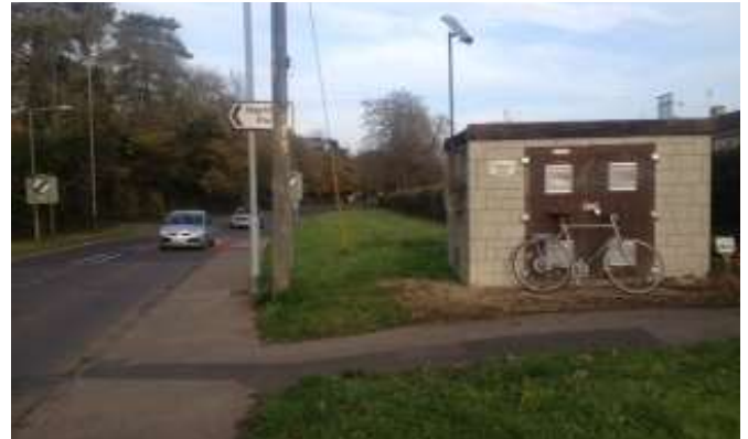
Sub station on the A4 - a candidate for screening?
