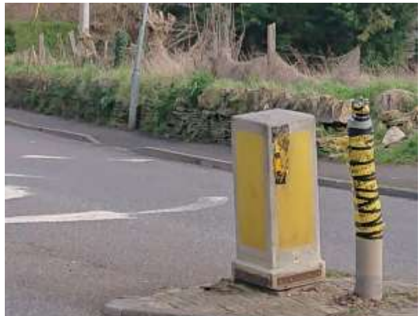
Damaged street furniture at Academy Drive
