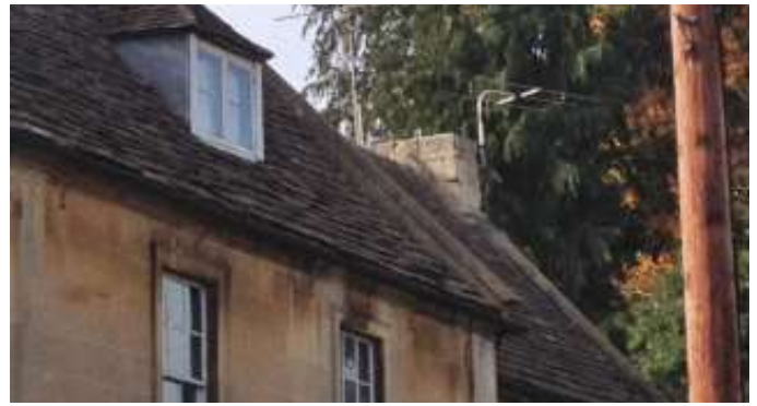
Chimney stump—at far end
