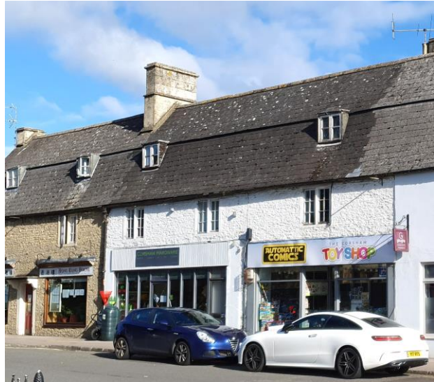
Above, Corsham Hardware, No. 27, which has been identified as the building in the photo. above left, on the basis of the arrangement of the dormer windows and chimney stack and the hood of what is now the Hong Kong House Chinese restaurant [far left].
