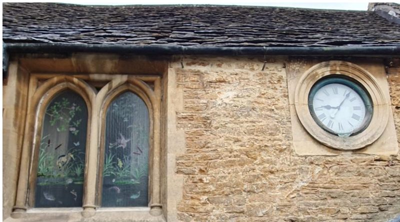
Above, the Thos. Bullock clock in the frontage wall of the Masonic Hall, Pickwick
